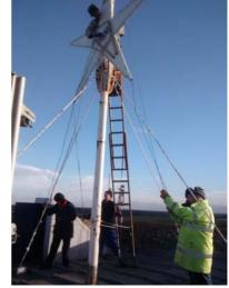
steady it until the clamps are fitted around the flagpole.
